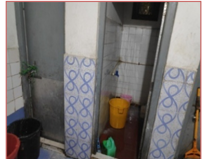
Damaged & Non-functional Toilets
